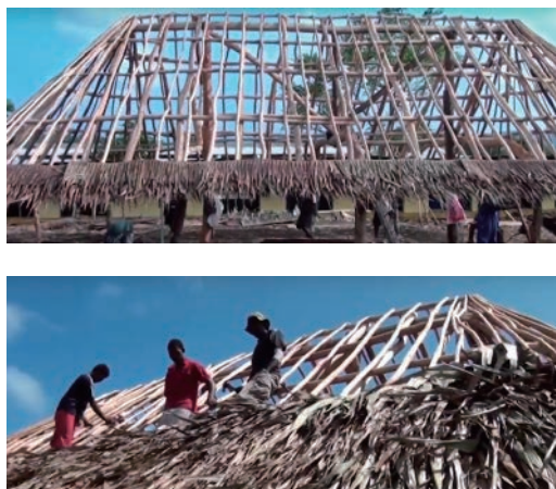
Figure 7 Lycee students constructing traditional house. (Source: Vanuatu Cultural Centre)
