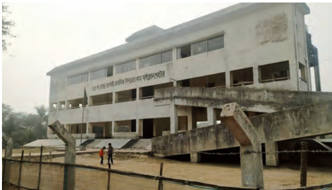
Figure 7 Cyclone shelter in Gabura (Photo: S.K. Abdullah Al Mamun)
